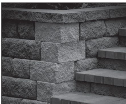
Outside 90-Degree Corner with Corner/Column Unit
