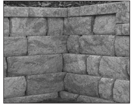
Example Inside 90-Degree Corner
