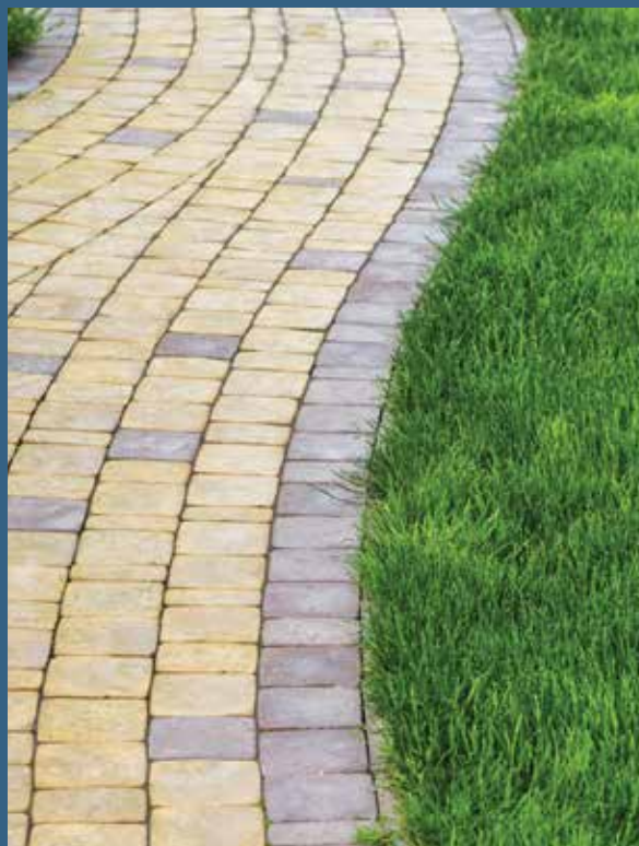
Correct Installation - Standard Edging
